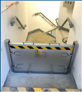
Single panel floodgate installed at staircase entrance of switch room
