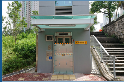
Two layer panel floodgate installed at Highway lift shaft
